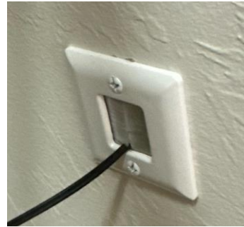
Into storage room (1st floor)
